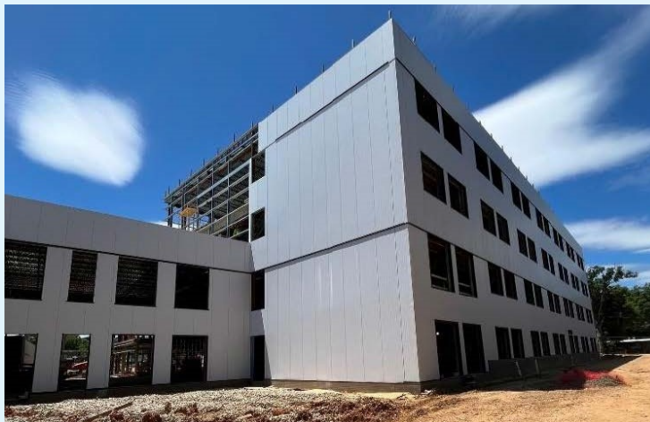
The new Hyattsville Middle School under construction
