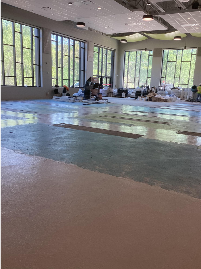
Cafeteria Terrazzo Installation
