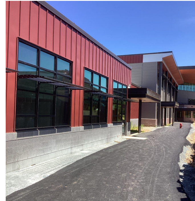
Temporary Walkway to Entrance of School
