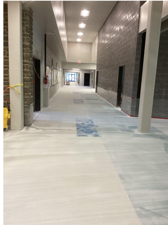
Ongoing Corridor Terrazzo Installation
