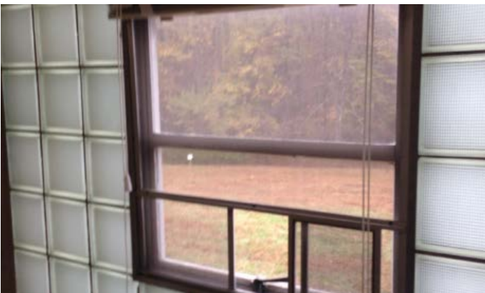
Orme Building: Glass block Wall
