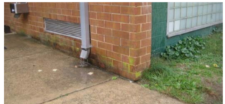
Orme Building: Roof Drains
