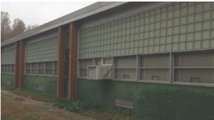
Orme Building: Exterior Walls
