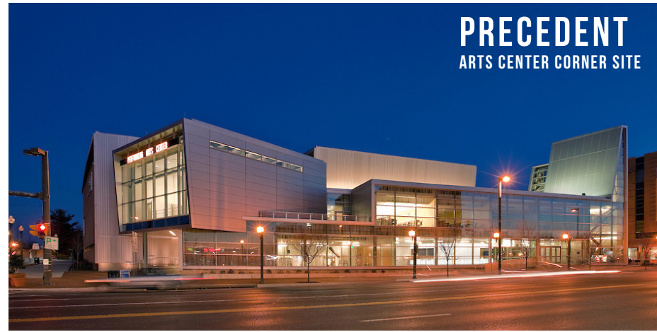
MONTGOMERY COLLEGE PERFORMING ARTS CENTER, SMITH GROUP
