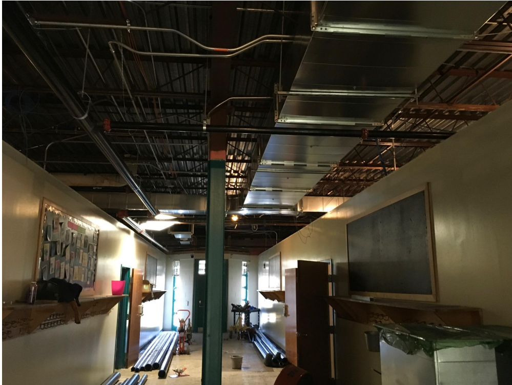
Newly installed ducts at POD A,B,C and D
