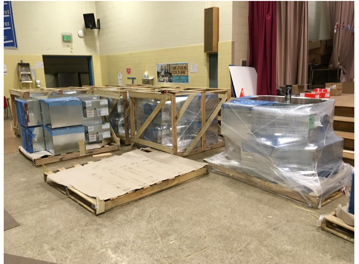
Other VAV's delivered and will be relocated to different rooms ready for installation.
