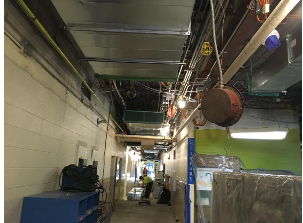
Newly installed duct at other areas of the building
