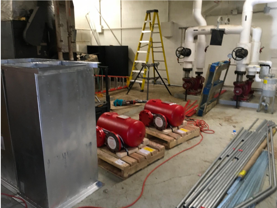
Boiler Room Existing Reciprocating Pump removal
