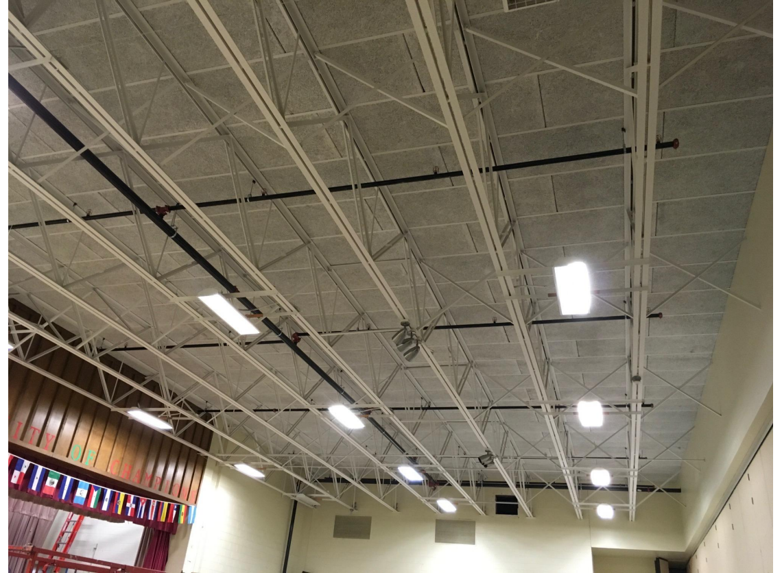
Other View of newly installed sprinkler pipes above Cafeteria
