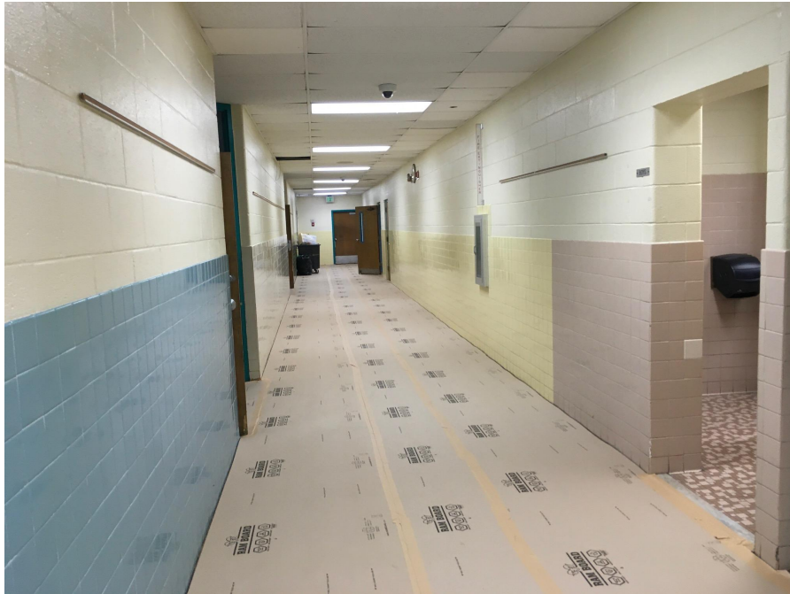
Protective Covering installed
