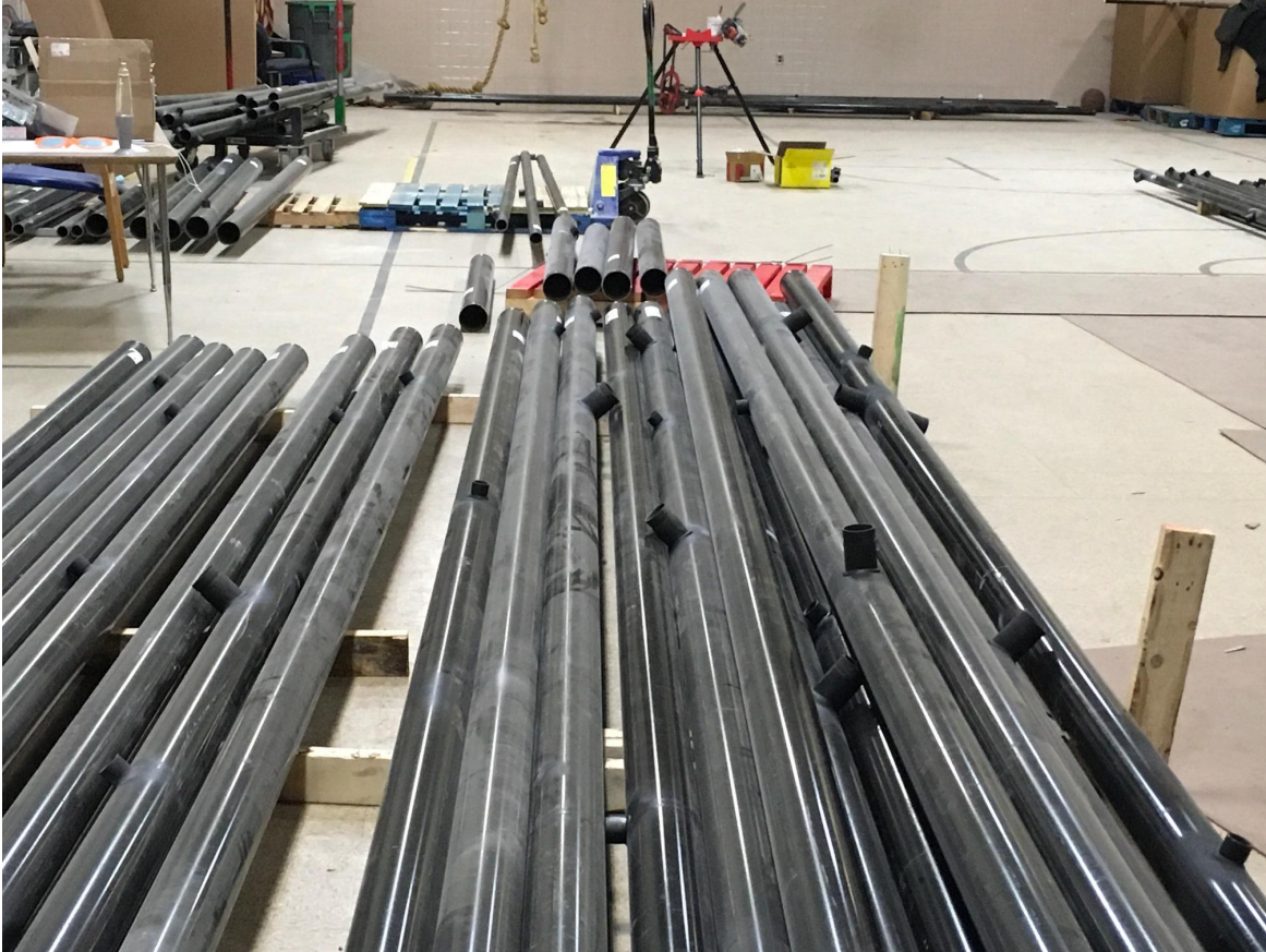
Sprinkler Pipes delivered and temporarily stored at the Gym
