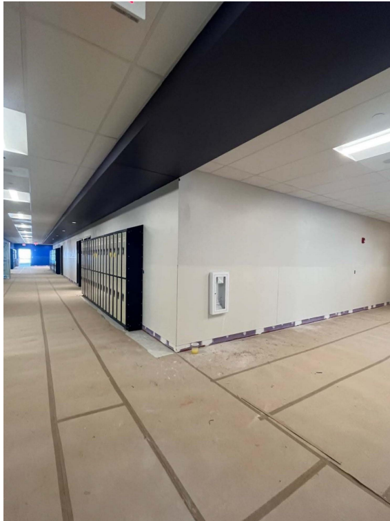
2nd Floor Corridor
